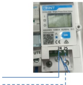
Figure 29 - ZSM-METER-DDSU Meter PIN Connections
