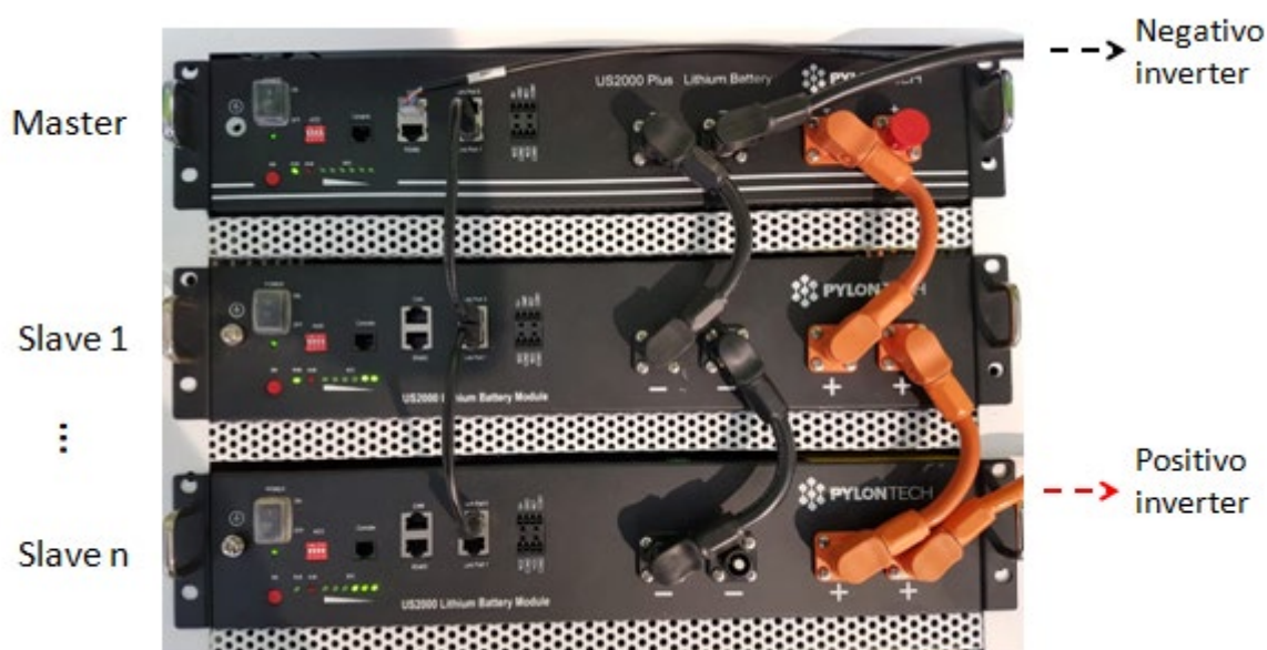
Figure 11 – Connecting three Pylontech batteries in parallel
