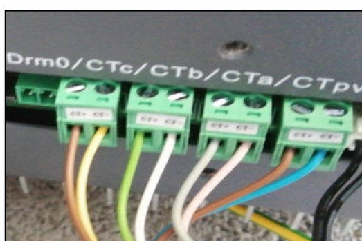
Figure 79 – Connecting the CT cables for the current sensors
