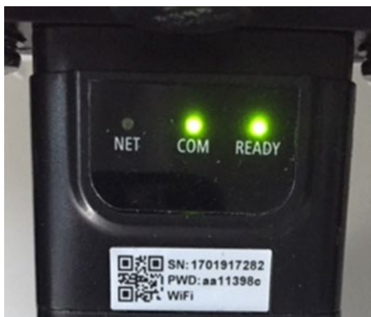
Figure 74 - Irregular communication status between the adapter and remote server
