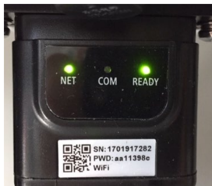
Figure 109 - Irregular communication status between inverter and adapter
