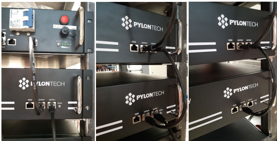
Figure 31 - Communication connections: The BMS and the first battery module (left), connection between the battery modules (centre), connection between the second-last and last battery module in the series (right)
