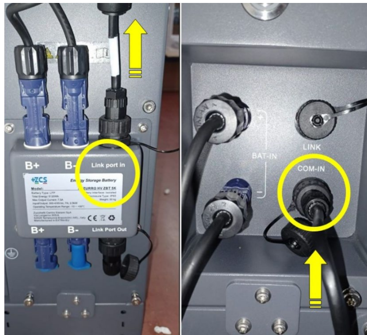
Figure 116 - Communication connections: BDU and first battery module
